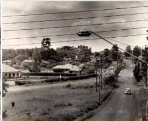
Lower Kabete Road between Malborough and Brookside Drive benefitted by the erection of 12 400 watt mercury lanterns of the Dioptron type.
